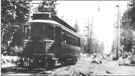
Figure X. Fourth Avenue Streetcar line freshly installed. Streetcars were provided before roads were improved or land subdivided for homes as a necessary precondition for development. Here is the scene a few years before these other urban features are built. Source: Vancouver: The Way it Was (Whitecap books)
